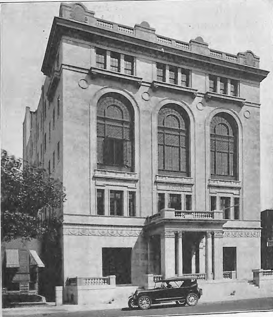
Elks Club Building, Jersey City, N. J. Wm. Neumann, Architect. This is one of many Lodge homes built of Indiana Limestone.
