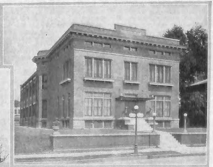
The new Home of Muscatine, Iowa, Lodge No. 304 was recently remodeled and redecored
