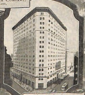
HANNA BUILDING ANNEX AND THEATRE Cleveland, Ohio Architect—C. A. PLATT, N. Y. Contractors—JOHN GILL & SON Cleveland, Ohio Russwin Dealer THE LUETKEMEYER CO.
