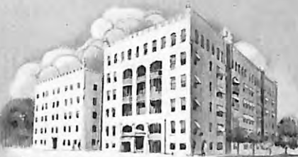
EMMONS APARTMENTS, HUNTINGTON, WEST VIRGINIA Architects—MEANOR & HANDLOSER Russwin Dealer—EMMONS-HAWKINS HARDWARE CO.
