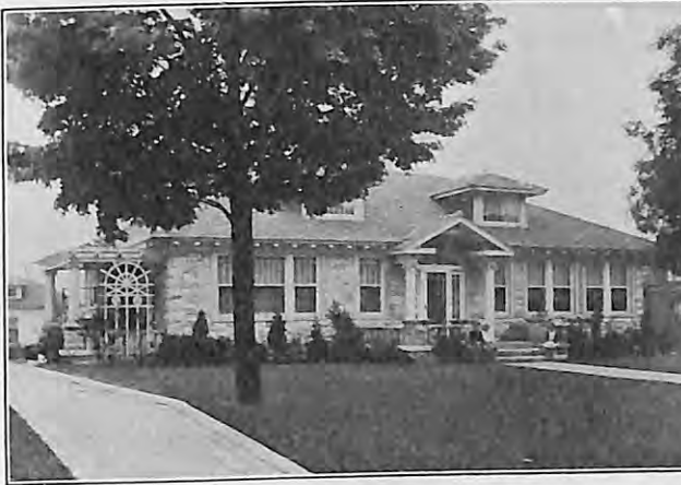
Design No. 401. Bungalow of seven rooms and bath. Faced with a veneer of Indiana Limestone having rough rock finish.
