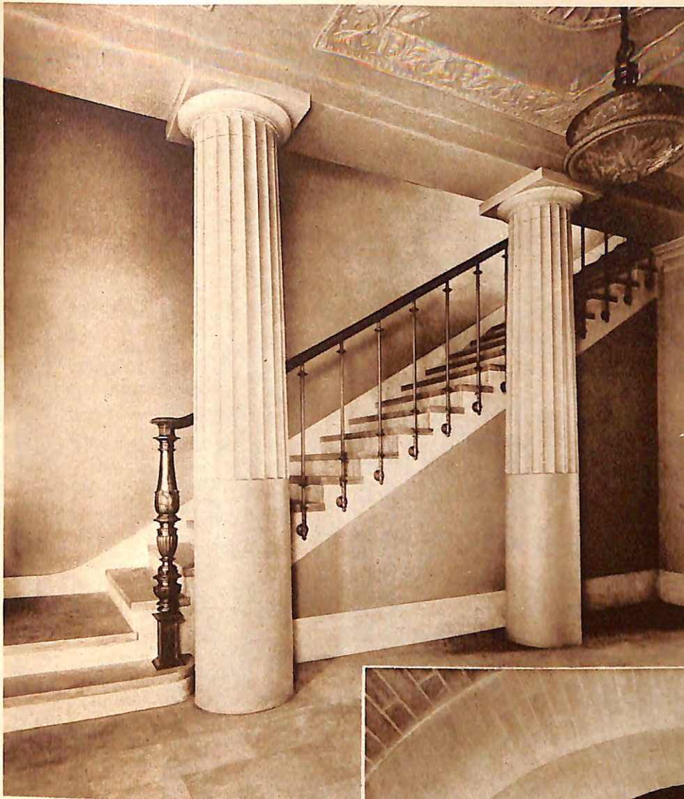
There is a stairway like this in each of the wings, leading up to the suites of offices on the second floor
