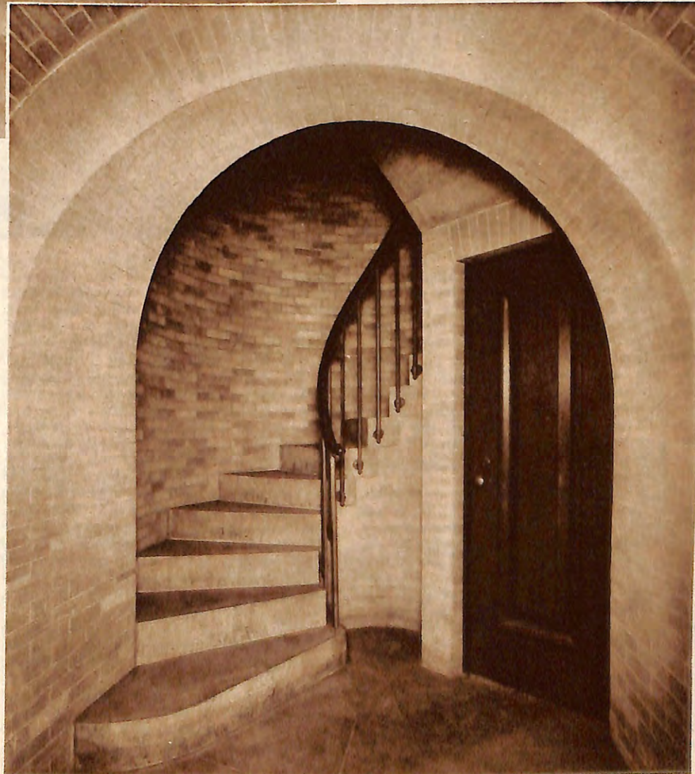
Below is the unusual brick spiral stairway leading to the outer colonnade
