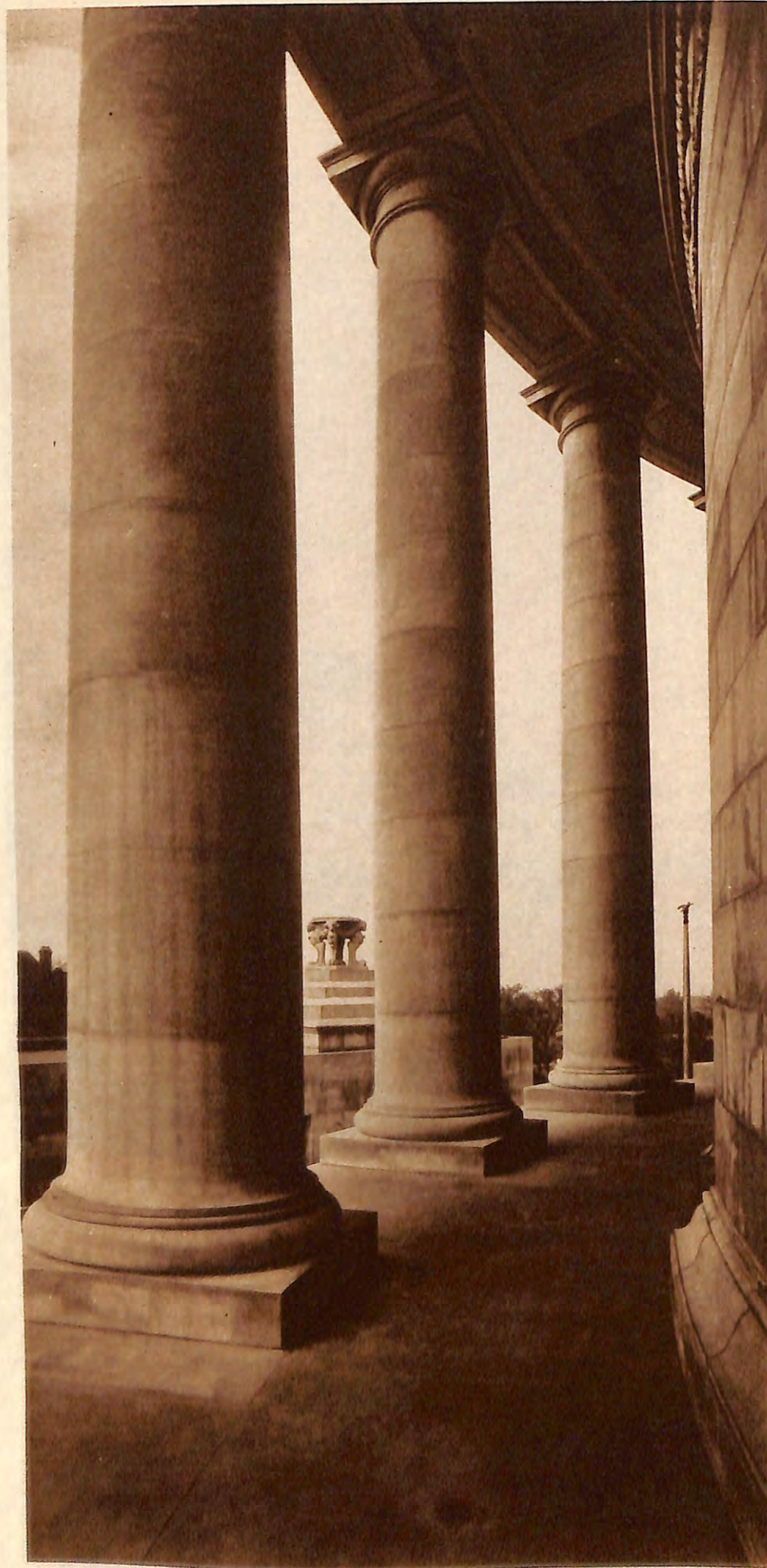
The majestic outer columns of the Memorial Hall. They are four feet thick at the base and thirty-two feet high. The urn is on the north wing
