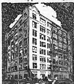
The Chicago factory of Harvey Bros. where all clothes are made in light, airy shops, operated under the most modern conditions. A tailoring staff with thirty years experience, and four million dollars backing turn out garments that are guaranteed to the utmost.
