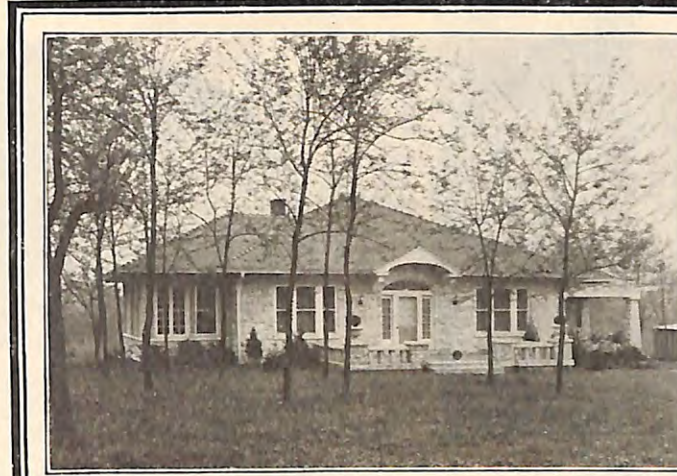
Design No. 403. Bungalow of eight rooms and bath, with both open and covered porches. Faced with a veneer of Indiana Limestone having rough rock finish.
