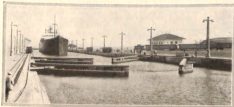
Should anything go amiss at Gatun Lock, instant communication with every point on the Panama Canal can be established through telephones concealed in the light pillars
