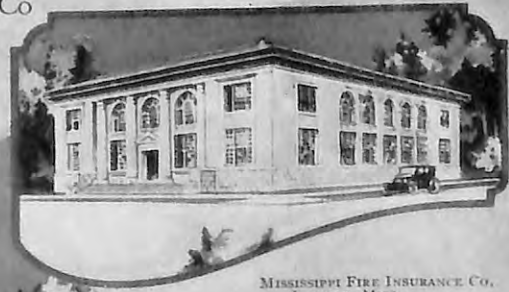
MISSISSIPPI FIRE INSURANCE CO., JACKSON, MISS. Architect —N. W. OVERSTREET, BIRMINGHAM, ALA. Contractors —E. G. PARRISH CONSTRUCTION CO., JACKSON, TENN. Russwin Dealers —JACKSON HARDWARE CO., JACKSON, MISS.
