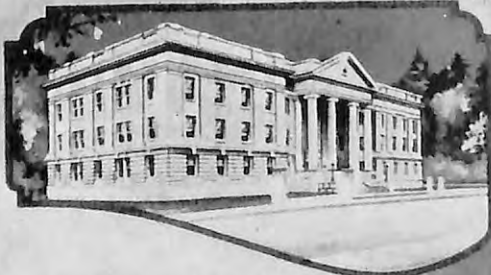
SKAGIT COUNTY COURT HOUSE, MT. VERNON, WASH. Architect —F. F. DOAN, BELLINGHAM, WASH. Contractors —ALEXANDER & MACNEIL, MT. VERNON, WASH. Russwin Dealers —MORSE HARDWARE CO., BELLINGHAM, WASH.
