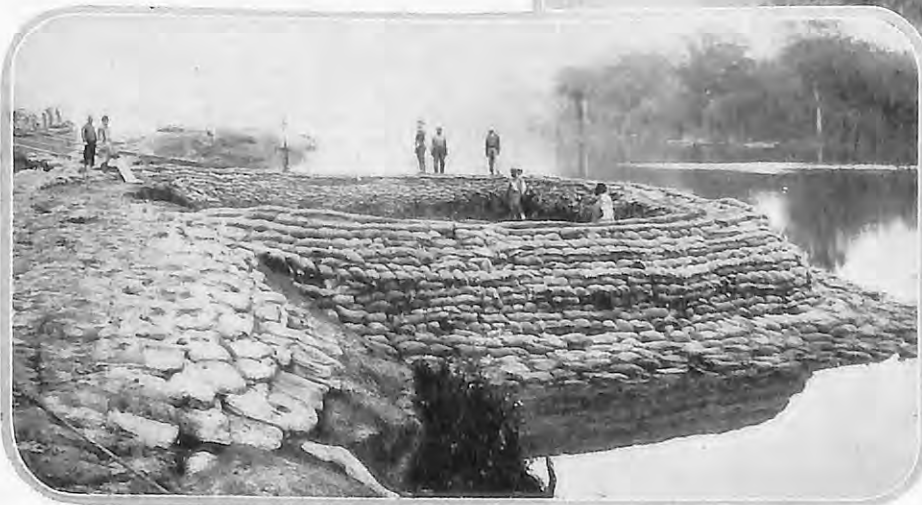
Here you see (below) how the sandbags are piled on the levee tops against the gnawing action of waves
