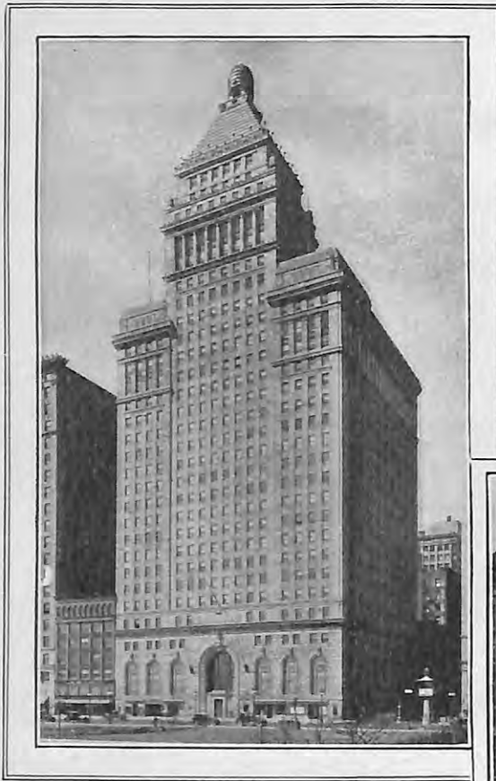
Both the Chicago and New York Straus buildings are of Indiana Limestone. At the left is the Straus Building on Michigan Boulevard, Chicago. Below is the New York building.
