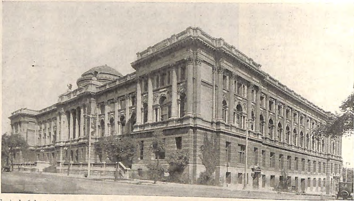
Typical of the city's magnificent buildings is this one. It houses the Milwaukee Public Library and Public Museum
