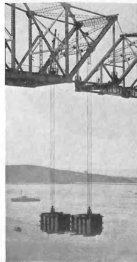
AMERICAN BRIDGE CO.
