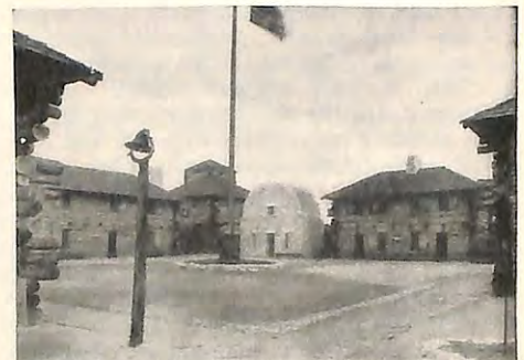
This replica of Old Fort Dearborn stands on the lake-shore at Twenty-sixth Street
