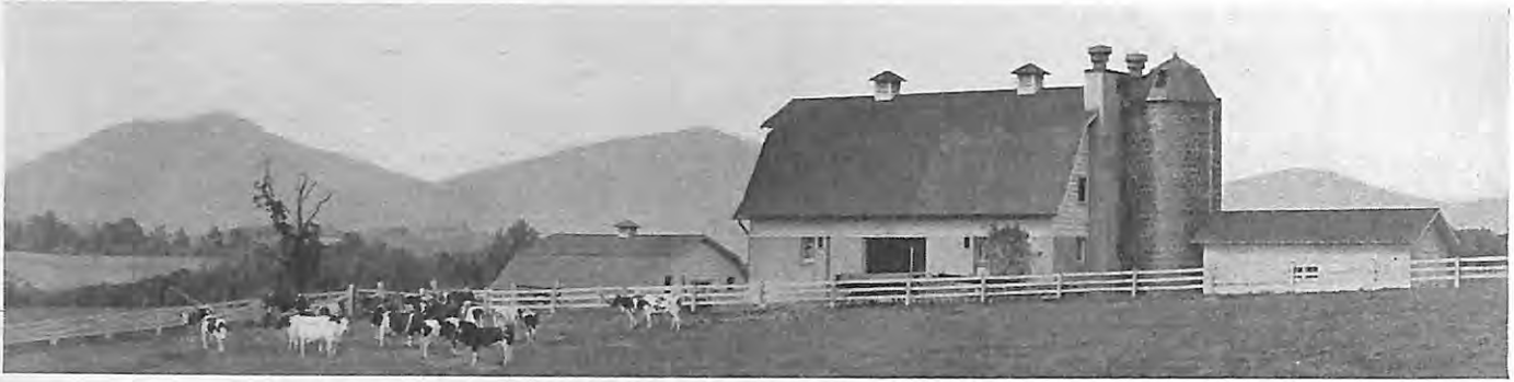
The up-to-date barns and silo at The Elks National Memorial Home at Bedford, Va.
