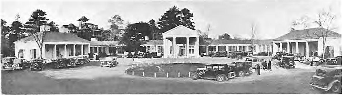
Georgia Hall, Warm Springs Foundation, built by popular subscription of Georgia's citizens and recently dedicated by President Roosevelt
