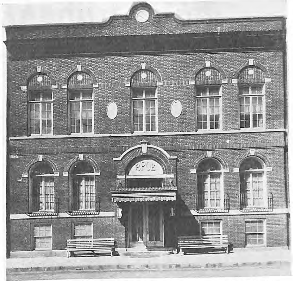
The new Home of Martinsburg, W. Va., Lodge, where the West Virginia State Elks Association Convention will be held August 12, 13, 14
