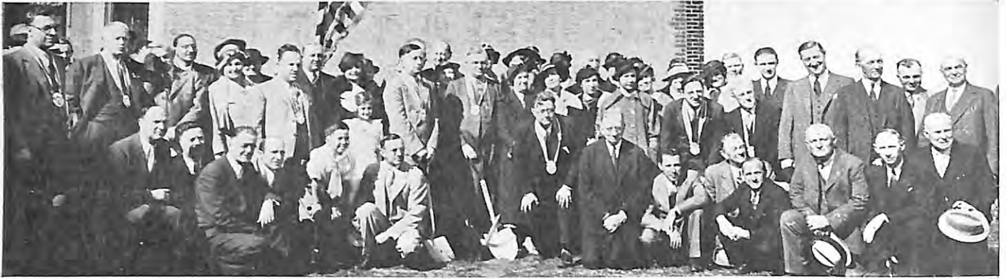
Distinguished officers and members of Weehawken, N. J., Lodge breaking ground for the large and handsome addition to their Lodge Home. Many ladies attended the ceremonies
