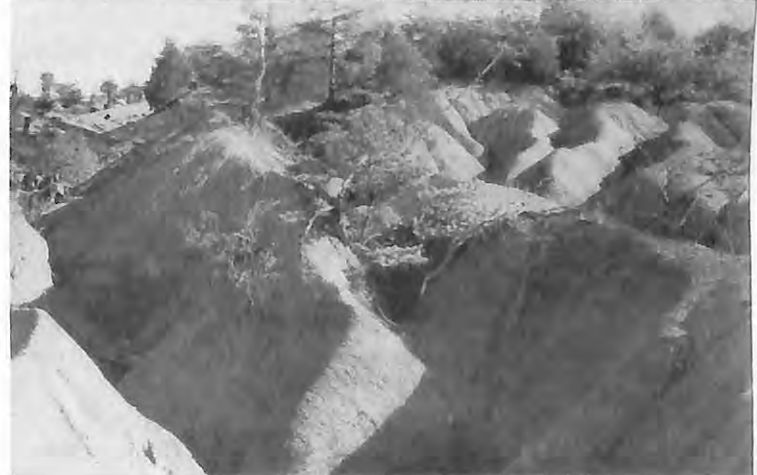
Above. A badly eroded hillside before the C.C.C. work began. When areas are deforested and water uncontrolled, this is what farmers can expect. Naturally, such land is totally unproductive.
