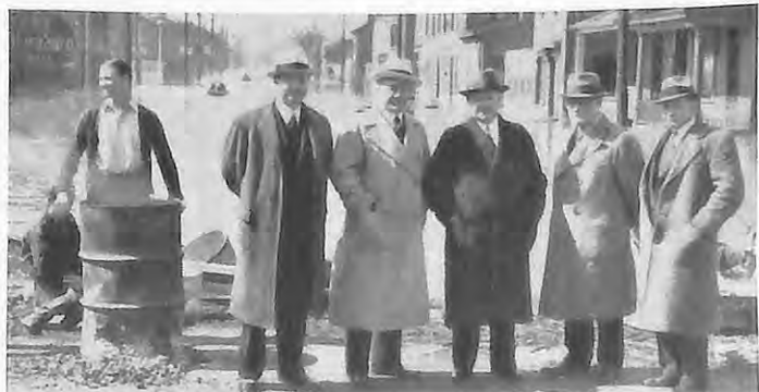
Grand Exalted Ruler Hallinan, with D.D. Charles B. Truesdell, of Kentucky, at extreme left, inspecting flood conditions on the occasion of the Grand Exalted Ruler's visit to Northern Kentucky
