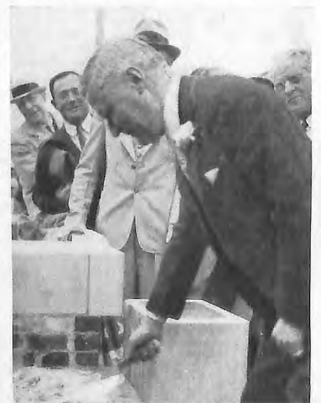
Below: Senator A. Harry Moore laying the cornerstone for the Therapeutic Pool at the Betty Bacharach Home near Atlantic City.
