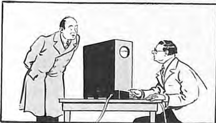
5. Just warming to his task, my guide said, "Here is the electro-magnetic tester that 'sees' through steel. It reveals hidden flaws in steel, much as the X-ray reveals broken bones in the human body."
