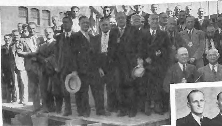
Officers of Flagstaff, Ariz., Lodge laying the cornerstone of the city's new postoffice
