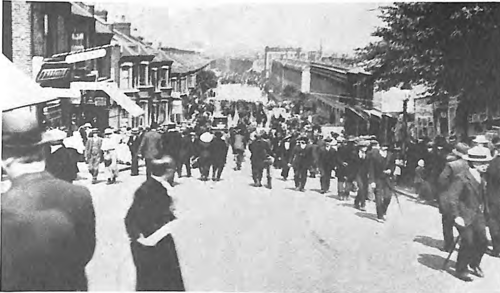
Above, a street in New Cross where much damage was done and many lives lost in a bad raid.
