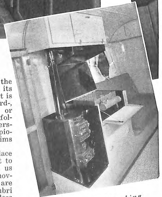
Heating and cooking equipment in the Silver Dome Hyway Coach
