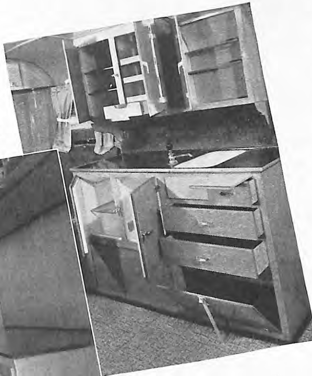
The compact and efficient ice-box, sink and cupboard units in, above, the Silver Dome Hyway Coach, and left, the Schult Trailer
