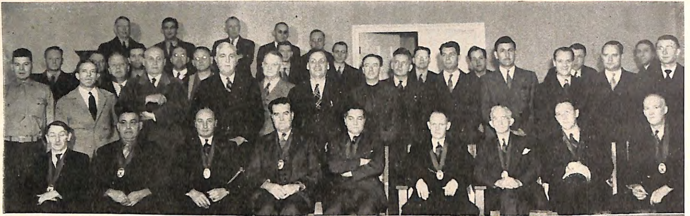
Above are members of Marshfield, Ore., Lodge, shown in their fire-scorched home. The small matter of a $10,000 fire did not stop the lodge from holding its regular meetings.
