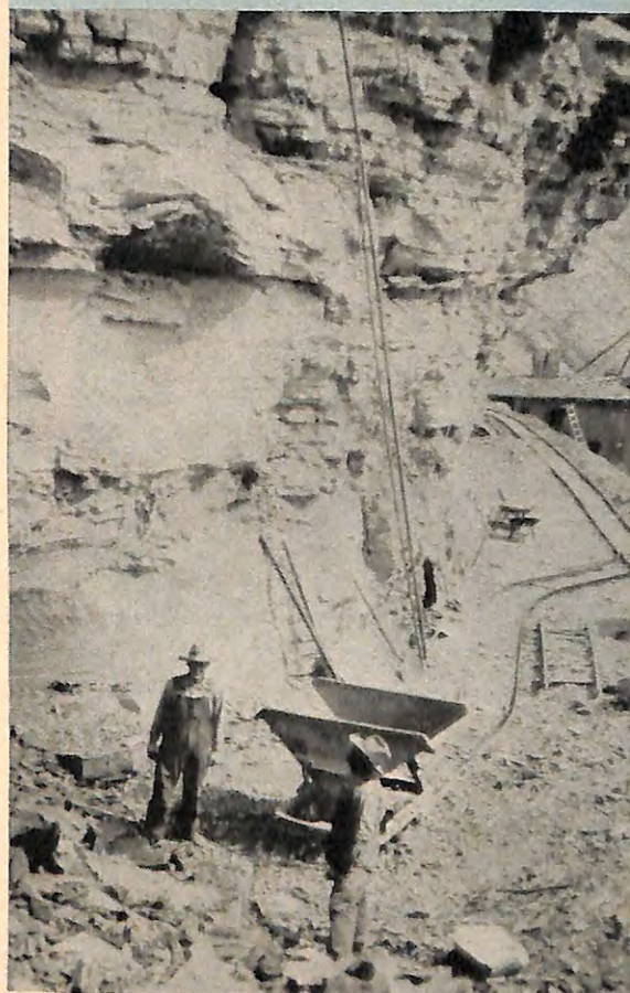
Oil shale quarrying operations at the old Bureau of Mines plant near De Beque, Colo. It is not practical to quarry oil shale commercially on such a small scale as this.
