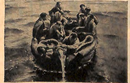
4 The outboard is mounted. Ample fuel is provided to swiftly power a good distance from enemy coast. Then motor can be quickly replaced with a collapsible rudder for use with sail.
