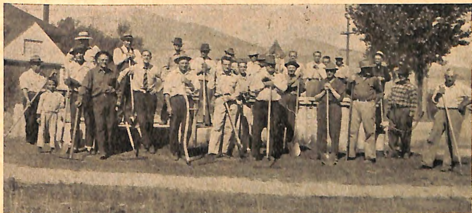
Left: Members of Hamilton, Mont., Lodge go to work cleaning up the lots where their new home will be located.
