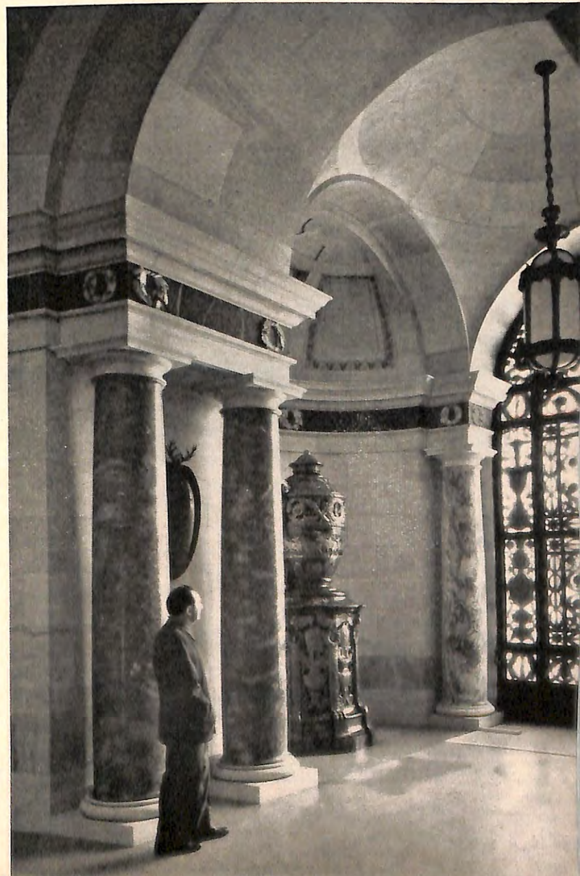
The massive carved bronze urns at main entrance in reality are screens for the radiators they conceal.
