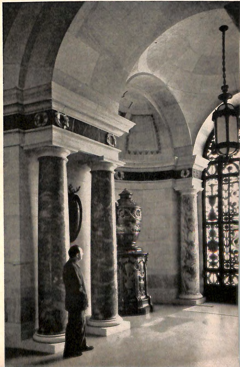
The massive carved bronze urns at main entrance in reality are screens for the radiators they conceal.
