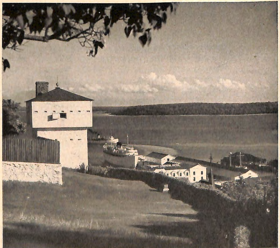
From Old Fort Mackinac on Mackinac Island. Blockhouse at left is a part of the Old Fort. Larger ship at the dock is the S.S. North American . Land in the immediate background is Bois Blanc Island and in the far distance is Michigan mainland.
