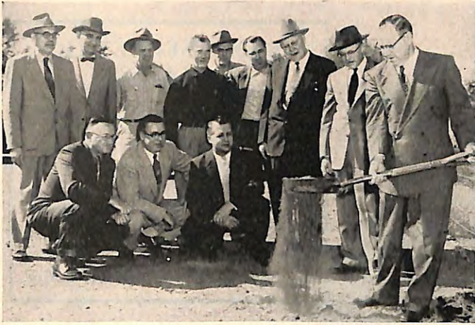
Bismarck, N. D., Lodge's Trustees Chairman Fred C. Hauser, in the presence of E.R. Glen H. Jahnke, Secy. J. J. Duffy, the Building Committee, other Trustees, the architect and contractor, breaks ground for the three-story office building the lodge is constructing on land it owns in the heart of the city, where a new lodge home will be erected.
