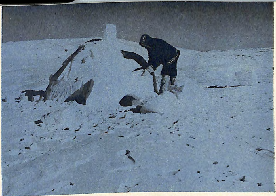
The Eskimos of the Canadian North build their igloos where hunting and fishing are found to be good. Blocks of snow with small pieces and loose snow filling the seams are arranged spirally by the Eskimos to form a chamber for living and then they cut and shape the entrance to the igloo.
