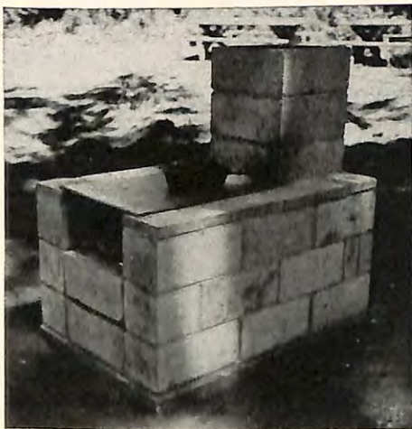
Made of concrete blocks, this fireplace (see figure 3) is a big, efficient unit for cooking.
