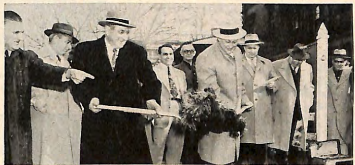
City Mgr. L. P. Cookingham assists E.R. Robert W. Boyle in breaking ground for the erection of Kansas City, Mo., Lodge's new home. The building, under construction for two months, will represent an investment of nearly $200,000 when it is completed and furnished.
