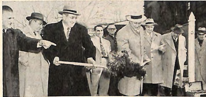
City Mgr. L. P. Cookingham assists E.R. Robert W. Boyle in breaking ground for the erection of Kansas City, Mo., Lodge's new home. The building, under construction for two months, will represent an investment of nearly $200,000 when it is completed and furnished.
