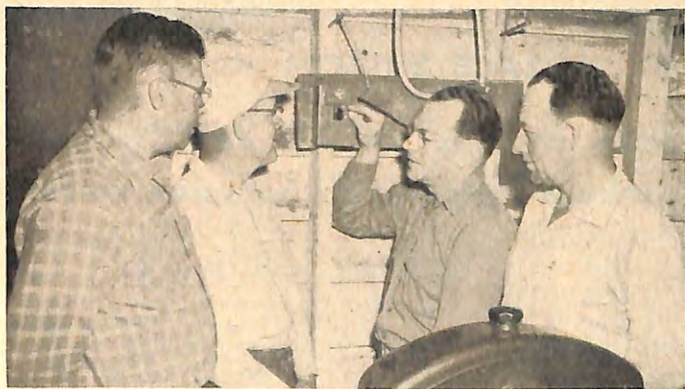
E.R. Earnest Heeb of Bozeman, Mont., Lodge throws the switch putting the Hyalite Youth Camp's new power plant into operation. At the dedication of this Elk project, made possible through the success of the lodge's Minstrel Show, were, left to right: Bill Sherwood, Dr. Wayne Thompson, President of the Camp Association, Mr. Heeb and Youth Activities Committee Chairman George Barrett.
