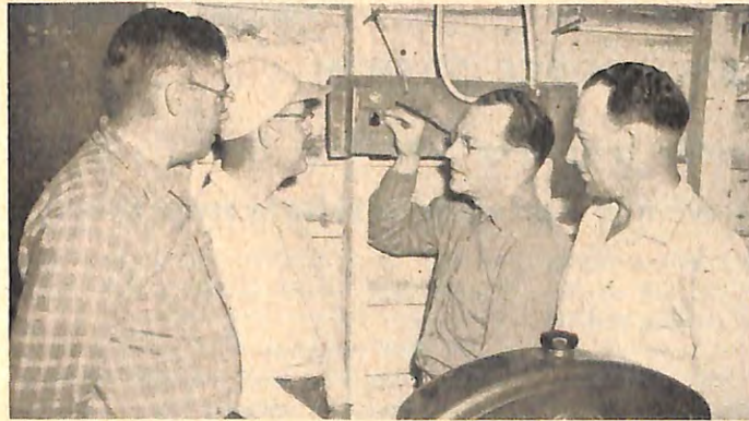
E.R. Earnest Heeb of Bozeman, Mont., Lodge throws the switch putting the Hyalite Youth Camp's new power plant into operation. At the dedication of this Elk project, made possible through the success of the lodge's Minstrel Show, were, left to right: Bill Sherwood, Dr. Wayne Thompson, President of the Camp Association, Mr. Heeb and Youth Activities Committee Chairman George Barrett.
