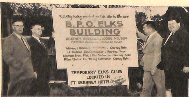
Kearney, Nebr., Lodge was in the process of building its new home when the Grand Exalted Ruler visited that city on October 20th. Photographed at the site of the new home were, left to right: Secretary R. A. Daugherty; H. L. Blackledge, member of the Grand Forum; Exalted Ruler Chester O. Marshall and Mr. Walker.
