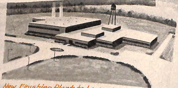
New Finishing Plant to be opened soon!
