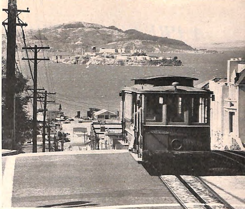
Cable car and Alcatraz Island in San Francisco Bay.
