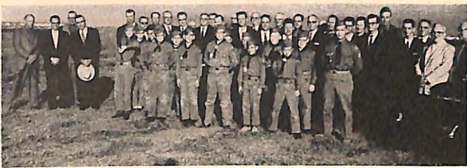
LUBBOCK, Texas, Lodge has broken ground for a $124,000 home. P.E.R. Hubert Griffin, a Trustee of the lodge and Chairman of the Building Committee, wielded the shovel; D.D. T. O. Wilkins delivered the principal address on this occasion; P.E.R. and Trustee Clyde Barger served as Master of Ceremonies; E.R. C. T. Richardson represented his Brother Elks, and Mrs. Clay Barger represented the Elks' ladies. Pictured with these participating officials is the Boy Scout Troop which the lodge sponsors.
