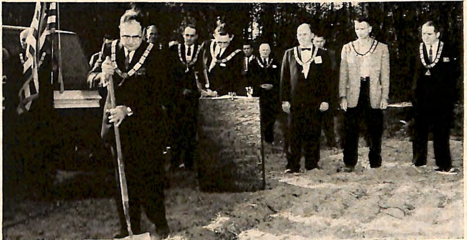
ARLINGTON-FAIRFAX, Virginia, Lodge's E.R. Herman C. Anderson breaks ground for a new $200,000 home in the presence of other lodge officials.
