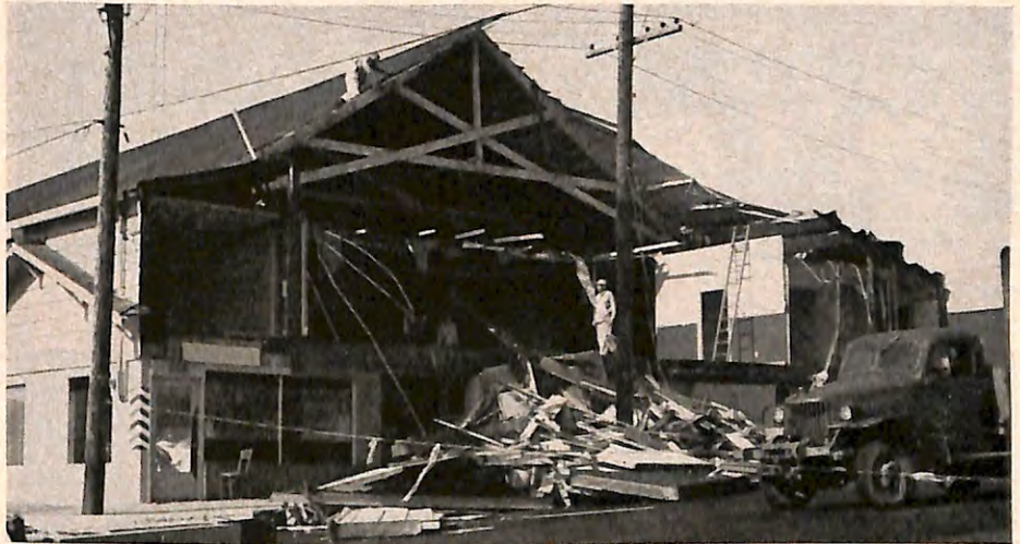
NEWPORT, Oregon, Lodge's home has a lean-to appearance since it suffered severe damage in the Columbus Day storm, the worst in 50 years. Business is going on as usual, however, with temporary cover protecting the damaged area.
