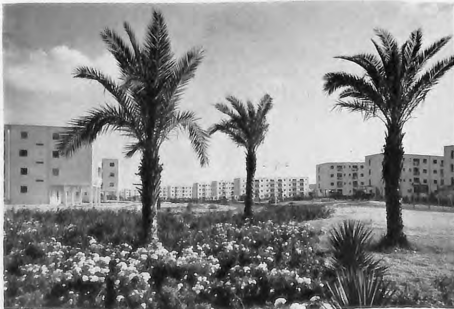
This government-sponsored apartment project in Holon, near Tel Aviv, indicates housing just doesn't "grow on trees" in the proverbial land of milk and honey.
