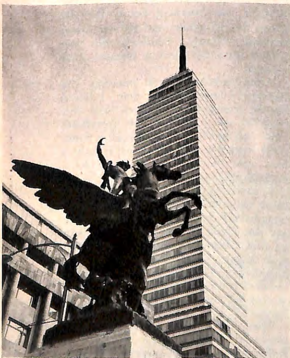
Mexico City's extreme altitude makes this 44-story modern structure the "highest" reaching building in North America.
