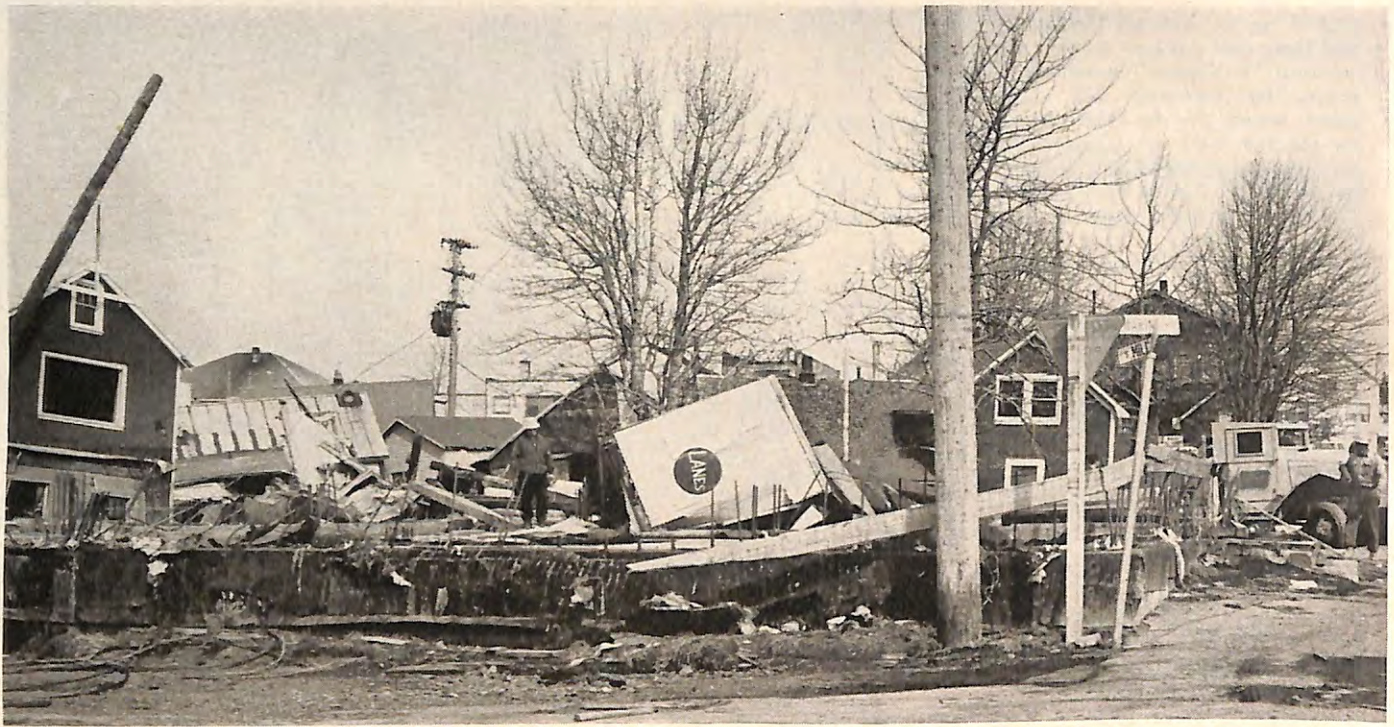
In the wake of the "tidal" wave which followed 'quake, the plan to use Kodiak Lodge's flooded bowling facility as the foundation for its new home is abandoned.
