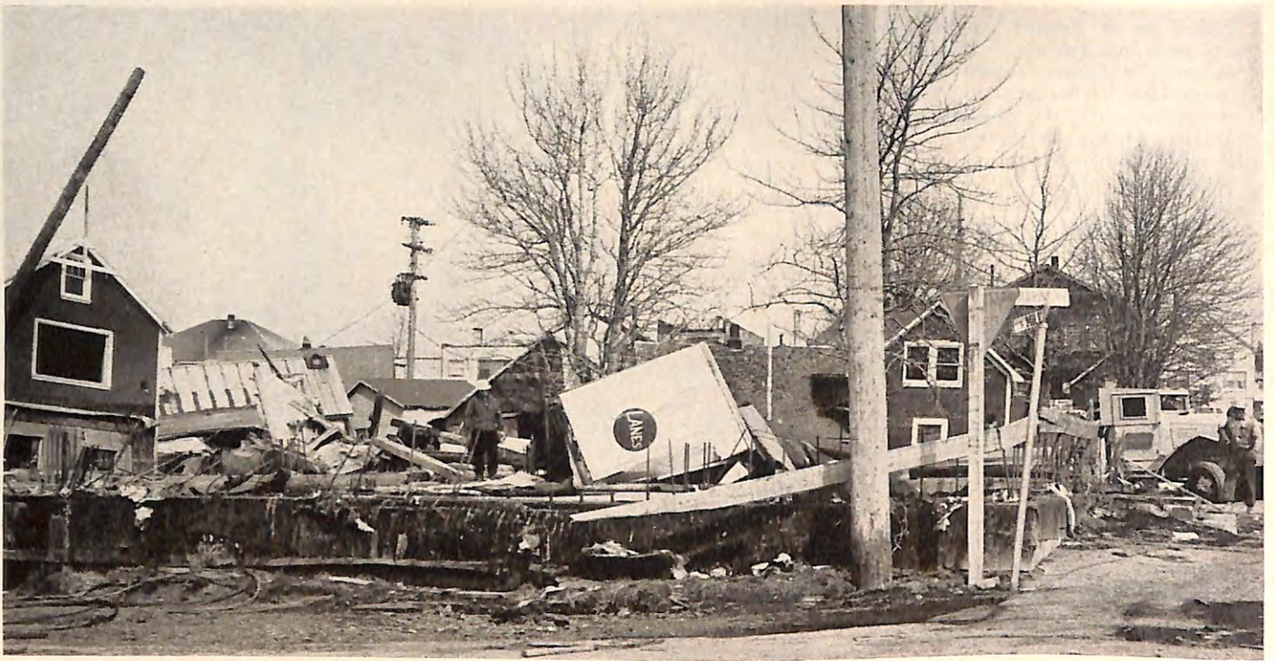
In the wake of the "tidal" wave which followed 'quake, the plan to use Kodiak Lodge's flooded bowling facility as the foundation for its new home is abandoned.
