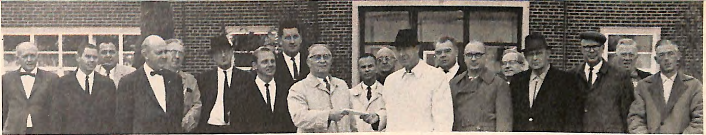
TRAVERSE CITY, Michigan, E.R. William Snelling, left center foreground, accepts the deed to the former Osteopathic Hospital from Director Lee Wyatt in the presence of other officers and the Lodge Building Committee. This building will be remodeled to replace the lodge home destroyed by fire a year ago.
