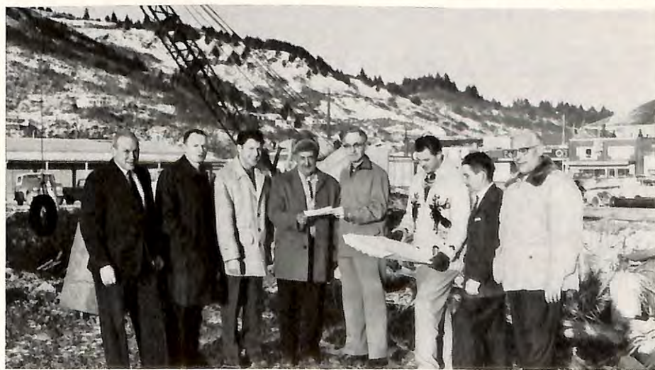
At the site of Kodiak Lodge's destroyed bowling alleys, members who are planning the rebuilding program look over architectural drawings. The buildings in the background are those remaining on Kodiak's main street; those on the other side of the street were heavily damaged and subsequently destroyed. Left to right
