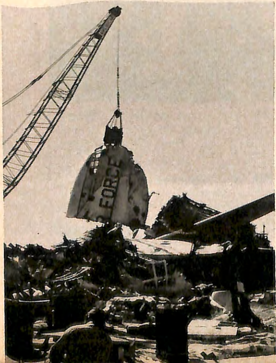
End of the line: The nose section of a KC-97 tanker-transport is plucked from a pile of scrap to be "guillotined" into sections, then fed into a furnace. Center, an entire tail section goes into the fire; right, metal ingots emerge from the other end. An entire KC-97 produces about 150 ingots for the scrap contractor who buys it.
