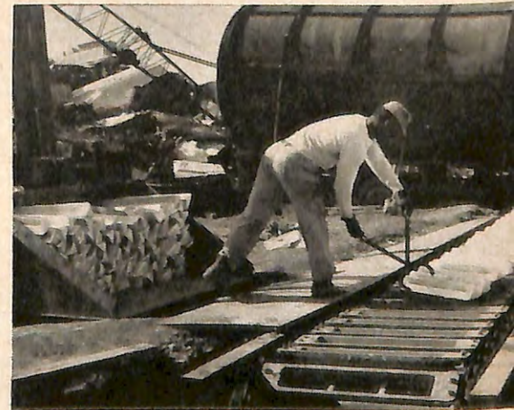
End of the line: The nose section of a KC-97 tanker-transport is plucked from a pile of scrap to be "guillotined" into sections, then fed into a furnace. Center, an entire tail section goes into the fire; right, metal ingots emerge from the other end. An entire KC-97 produces about 150 ingots for the scrap contractor who buys it.
